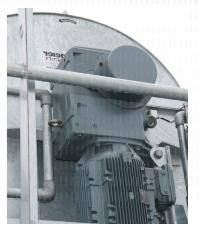
**Optimum operation** "The NORD drives are energyefficient. low-maintenance and robust to ensure reliable grain conveying at all times."
