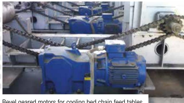
Bevel geared motors for cooling bed chain feed tables
